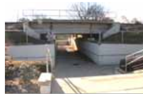
Grade-Separated Crossing Underpass
